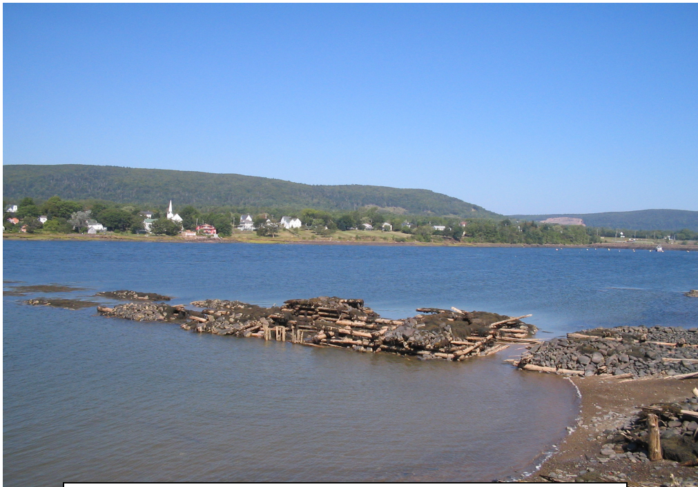
A low tide view of the remains of the Acadia Steamship Pier at the end of St George Street with Granville Ferry in the background. This pier once housed a spur of the Windsor and Annapolis rail line and an insulated apple warehouse.
